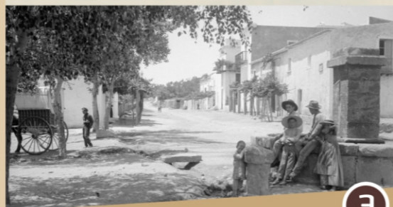
3 Es Broll i Pou de Baix The water pump and the Lower Well
